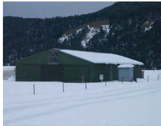
Nelson Lakes: Hangar
