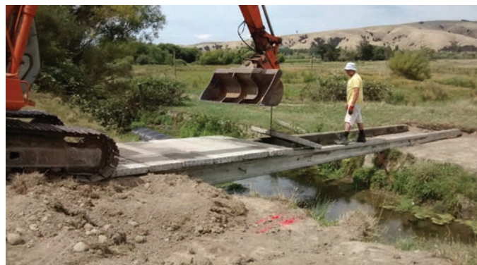
Bridge building Papawai Feb 16
