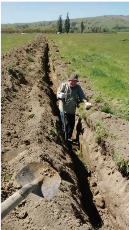
The power trench - Pressie Brian Sharpe Nov 15
