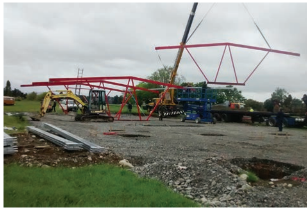
The hanger frame goes up Nov 15
