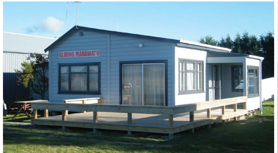
The club house almost finished.
