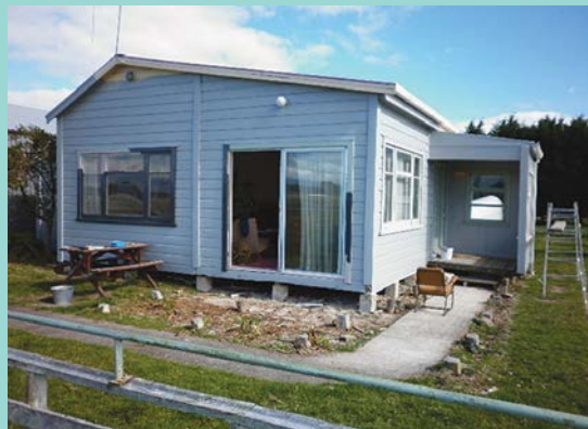
Painting done, Deck demolished in preparation for bigger and better version.
