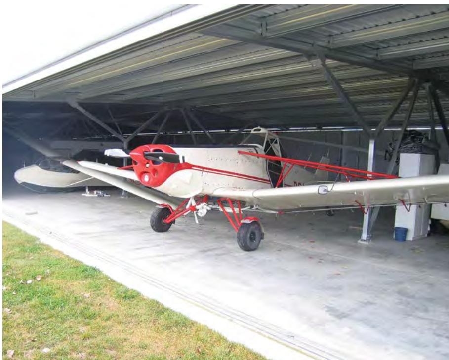
Photo –Southern Belle safely home in her new hangar at Omarama
